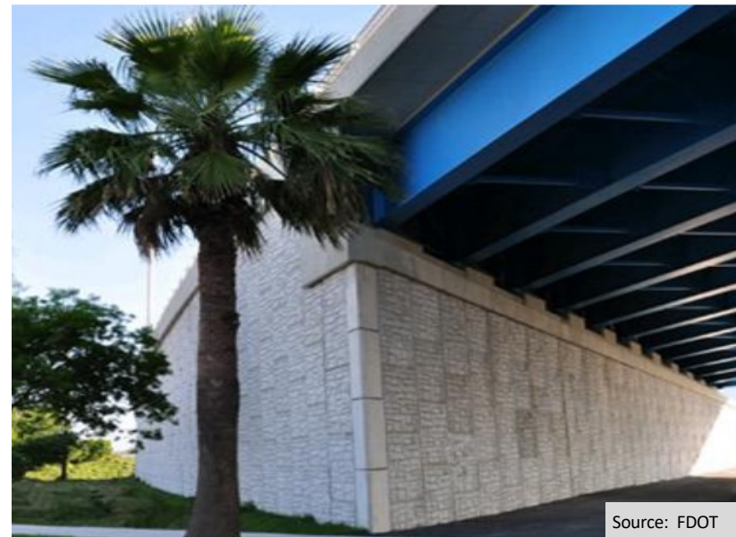
Example of Mechanically Stabilized Earth (MSE) Wall
